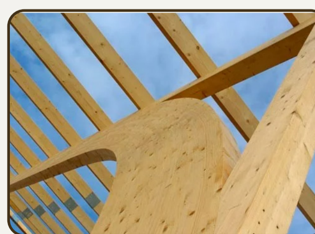
Glulam timber frame
