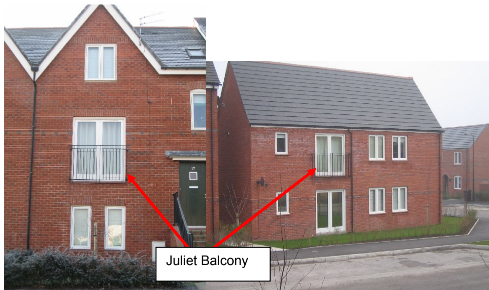
Figure 16 – Juliet Balconies in Completed Dwellings
