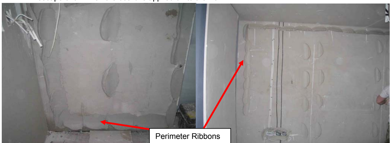
Figure 11 – Application of Perimeter Ribbons of Plasterboard Adhesive
