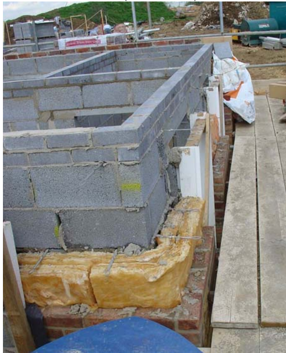
Figure 15 – Construction of Masonry Cavity Wall using Built-in Insulation (Site in Lincolnshire)
