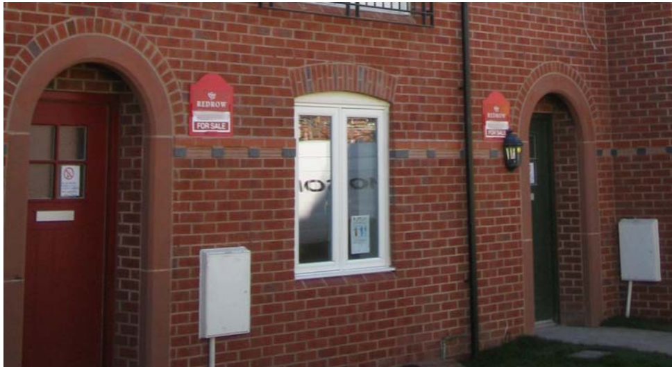
Figure 2 – Recessed Doors in Completed Dwellings
