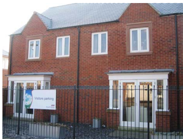
Figure 5 – Bay Windows in Completed Dwellings
