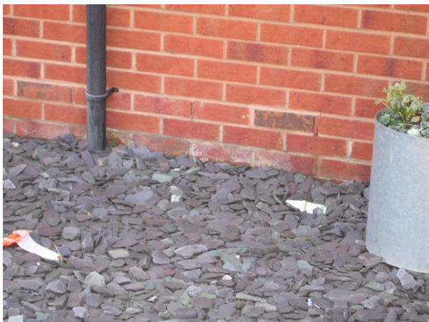
Figure 53 - Photograph and Thermal Image of External Wall-Ground Junction (One of the first dwellings to be constructed showing thermal bridging at slab edge – see paragraph 64)
