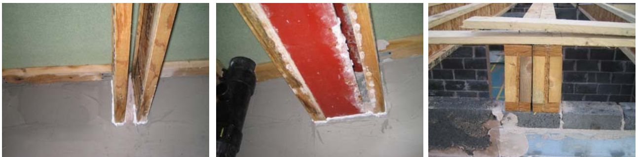
Figure 14 – Multiple Adjacent Built-in Joists and Beams
