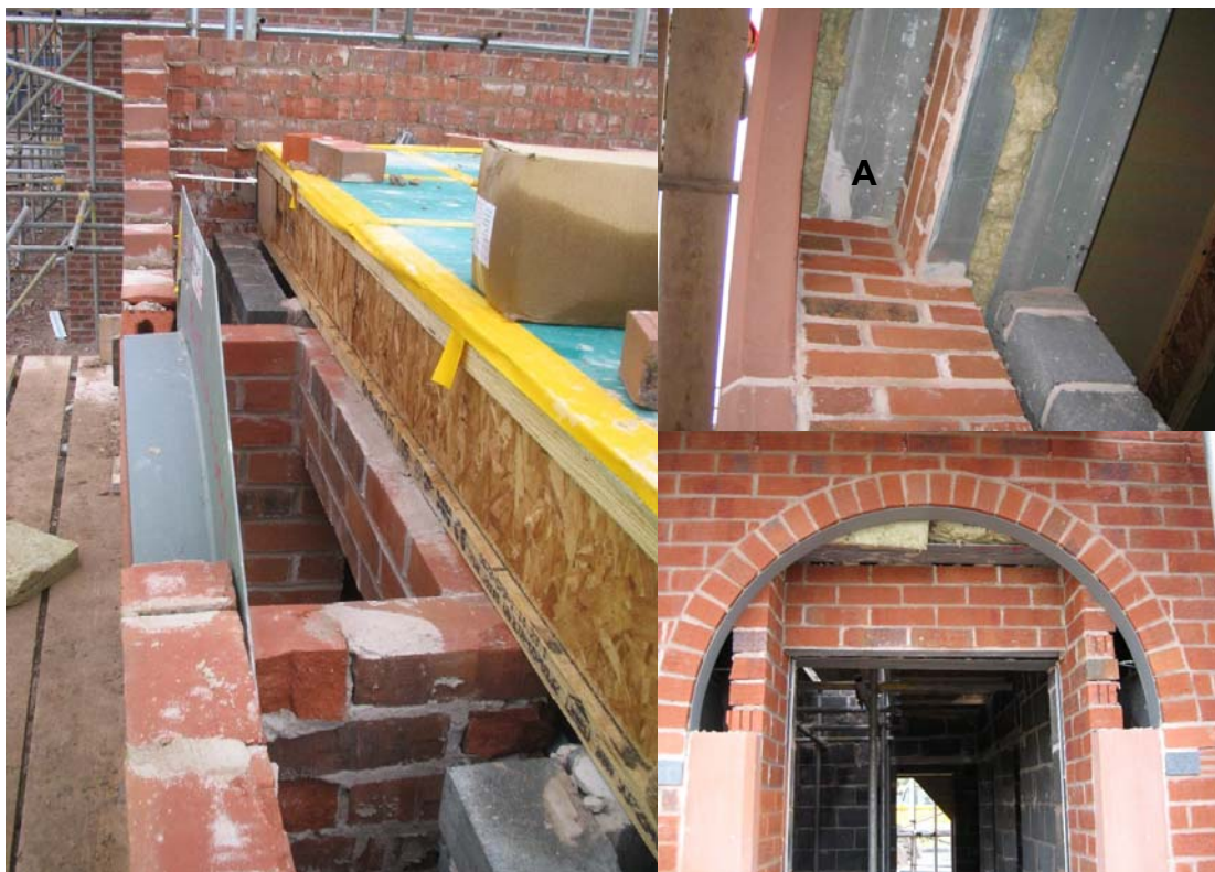
Figure 3 – Construction of Recessed Front Door
