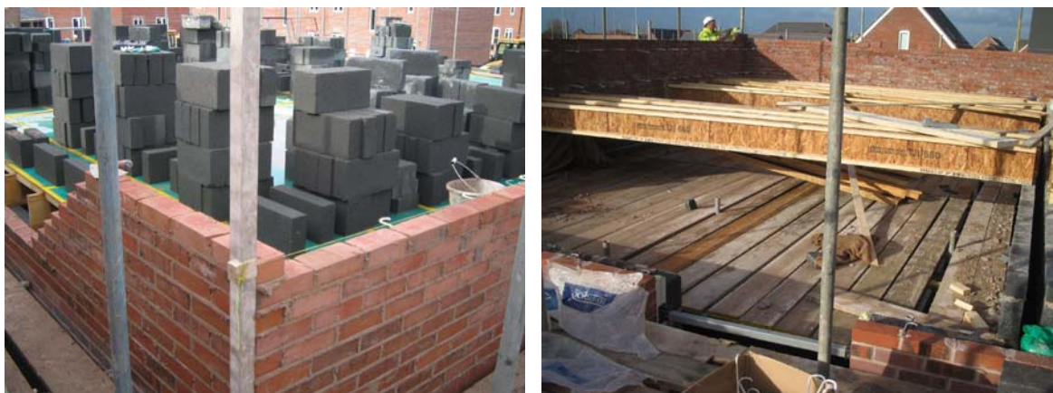
Figure 27 - Intermediate Floor Construction – External Leaf Built Before Inner Leaf
