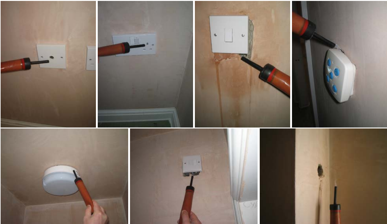
Figure 1.8 First floor electrical penetrations in all 3 bedrooms, landing, en-suite, cylinder cupboard and bathroom.
