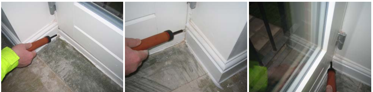
Figure 3.6 Leakage detected around the first floor patio doors in the master bedroom.
