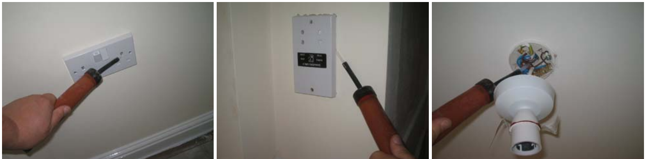
Figure 11.12 Movement of air through electrical penetrations on the 1 st floor on internal walls, service voids and into the ceiling.
