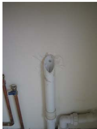
Figure 5.2 Temporary sealing of the washing machine waste pipe.
