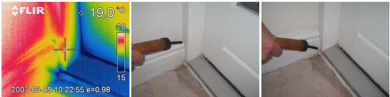
Figure 13.3 Ground floor patio door threshold.
