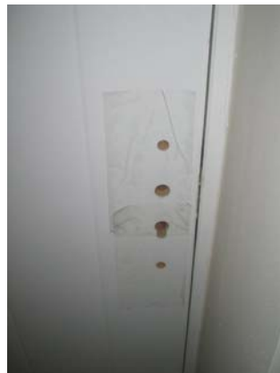
Figure 9.2 Temporary sealing to rear door.
