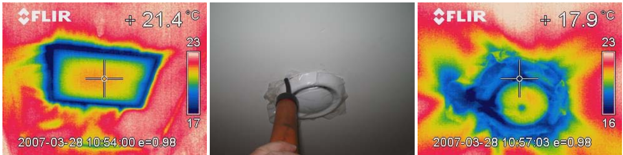
Figure 12.10 Air movement directly through the top floor ceiling.
