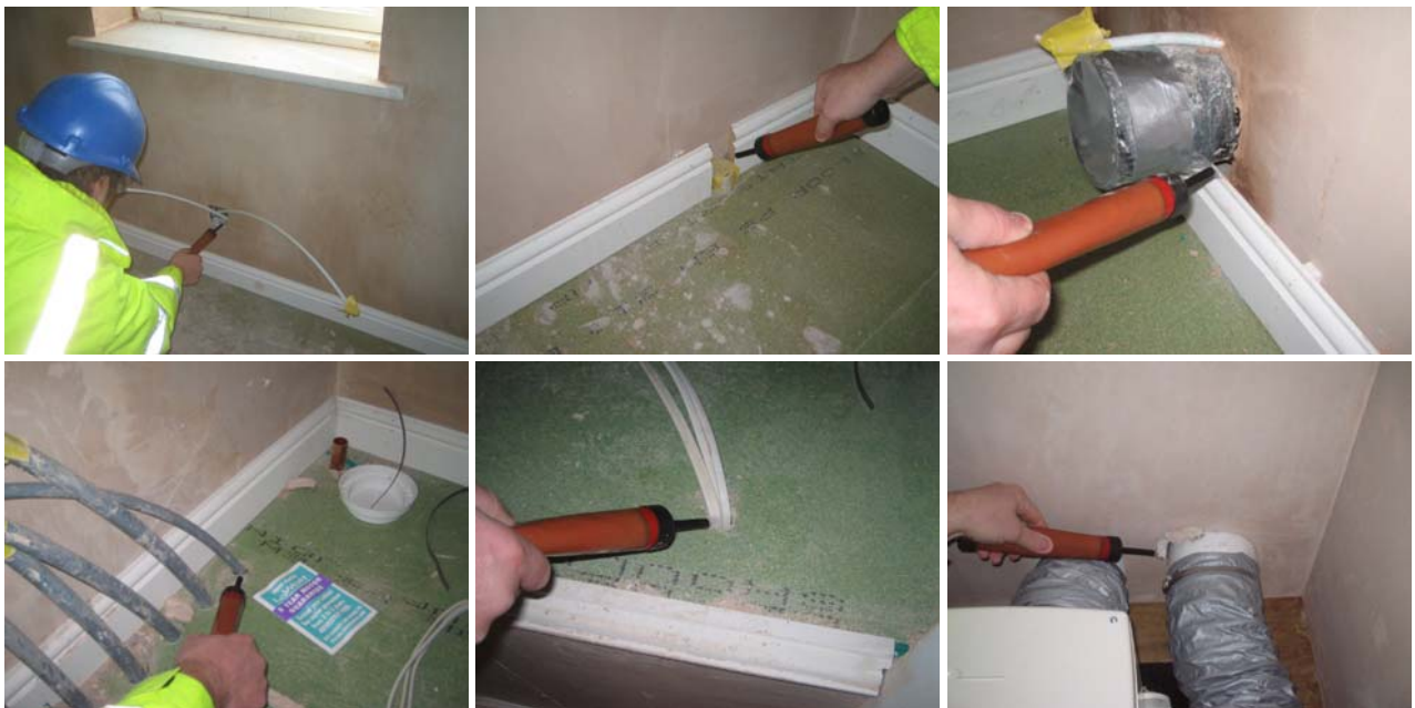
Figure 2.7 First floor plumbing penetrations
