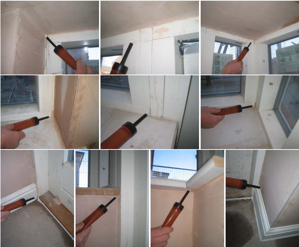
Figure 1.3 Air leakage around the bay window.
