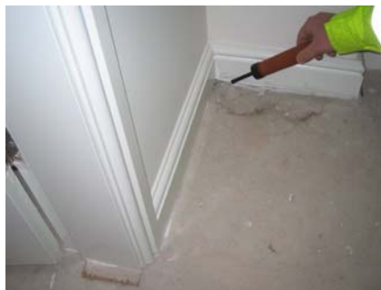
Figure 4.2 Ground floor perimeter in the utility room.
