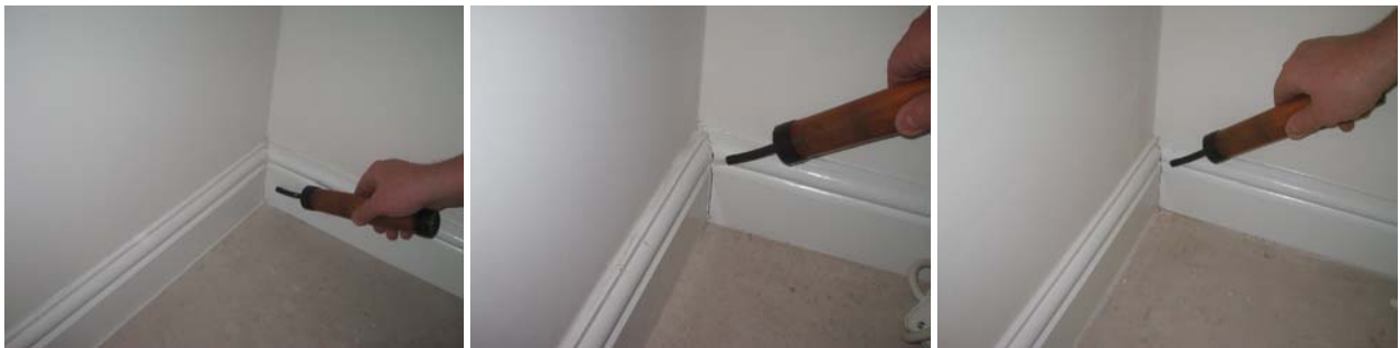
Figure 12.3 Air leakage at the ground floor skirting board junctions appeared more severe than when tested prior to the coheating test.
