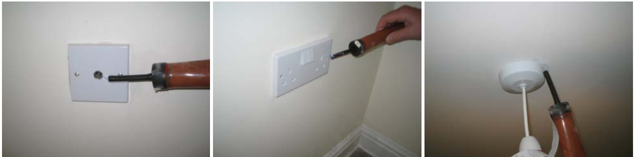
Figure 9.14 Air leakage at 1 st floor electrical penetrations at a bedroom aerial socket and through a power socket and lighting rose in the lounge.
