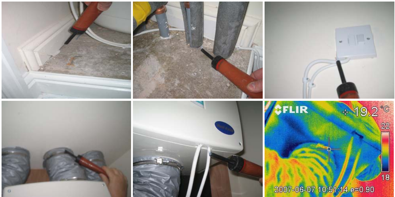
Figure 14.17 Air movement around junctions and penetrations in the 2 nd floor cylinder cupboard.
