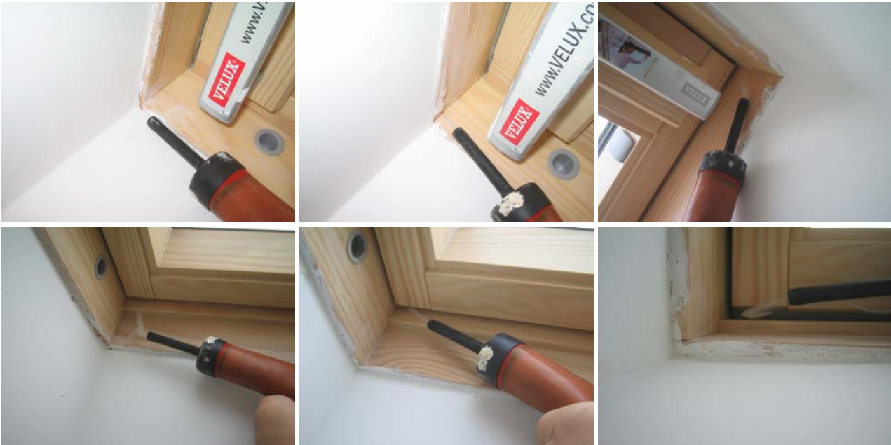
Figure 11.19 All 3 of the rooflights in the 2 nd floor rear bedroom displayed some degree of air leakage.
