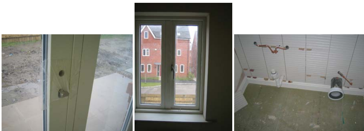
Figure 1.2 Temporary sealing prior to pressurisation test
