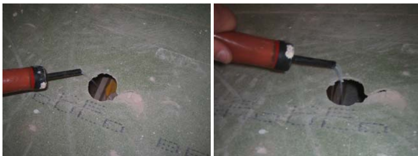
Figure 11.7 A hole in the 2 nd floor in the lounge allowing air to enter the floor void.
