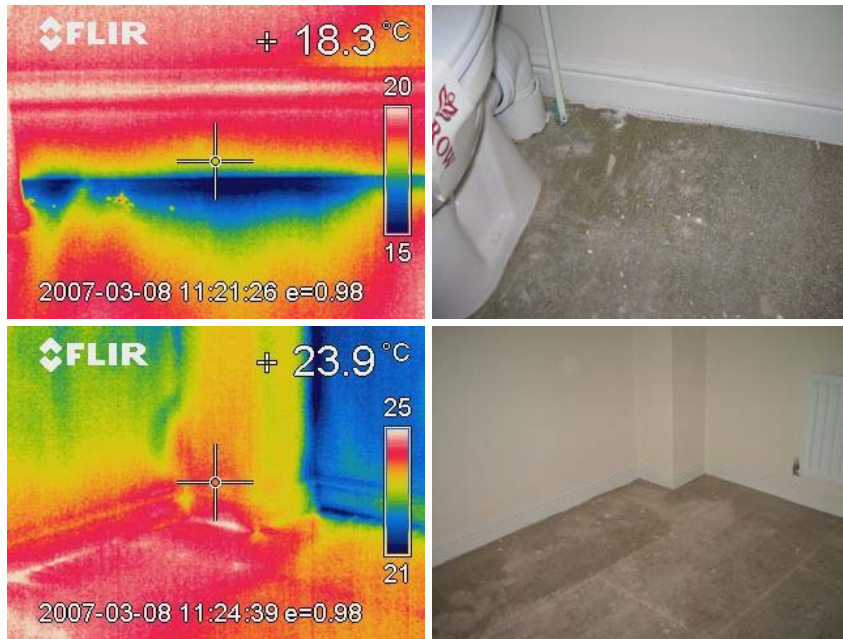
Figure 7.5 Air movement around the first floor perimeter; colder air entering at an external wall in the bathroom, and warm and cold air entering the rear bedroom on internal and external walls respectively.
