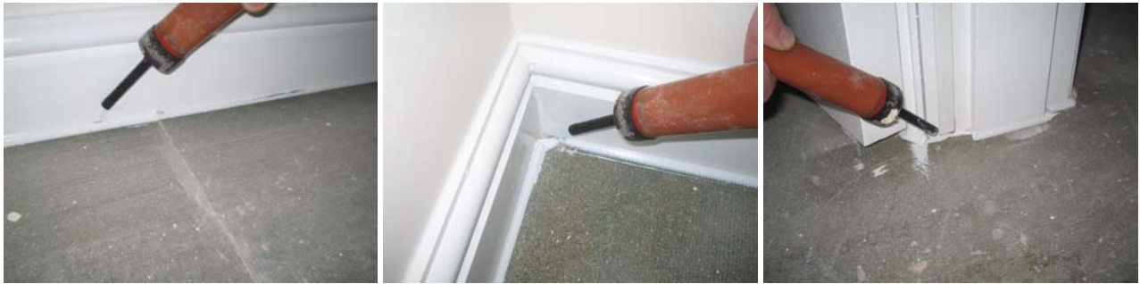
Figure 9.5 Air leakage was detected at gaps in the secondary sealing at the 1 st floor bedroom perimeters and the door between the lounge and landing.
