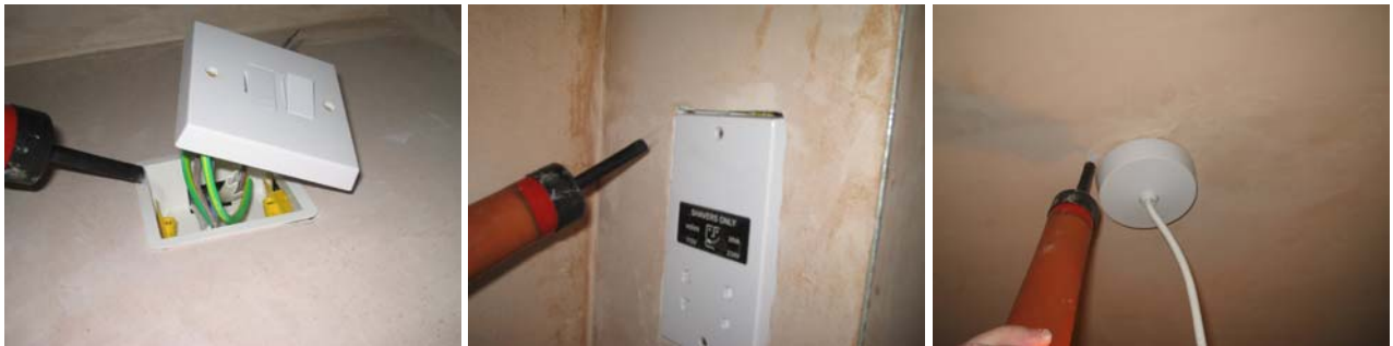
Figure 2.6 First floor electrical penetrations.
