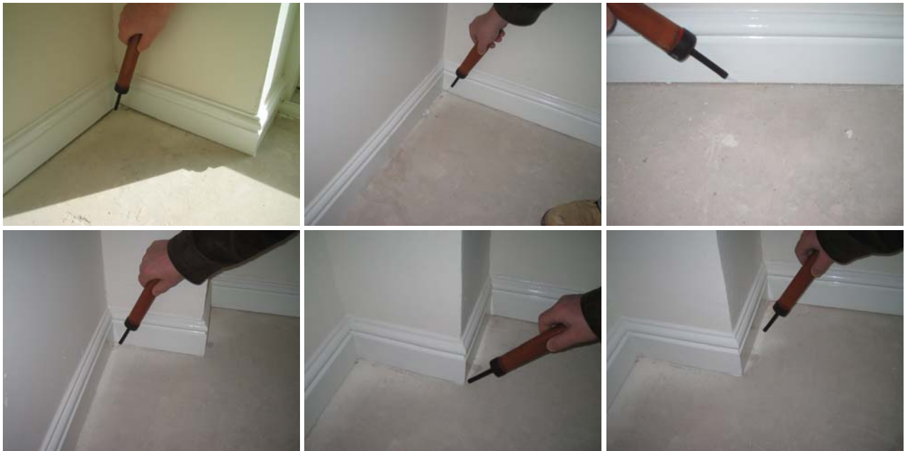
Figure 5.4 Air movement detected around the ground floor perimeter; on external walls in the kitchen, lounge and downstairs WC, and on internal walls in the lounge
