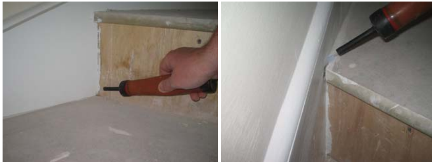
Figure 14.11 Air movement through gaps in the both staircases.
