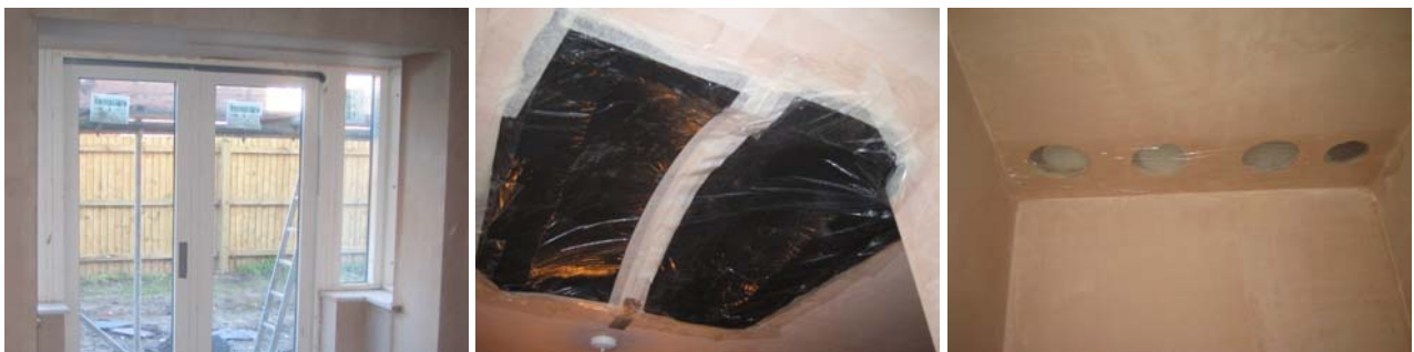
Figure 1.2 Temporary sealing prior to pressurisation test
