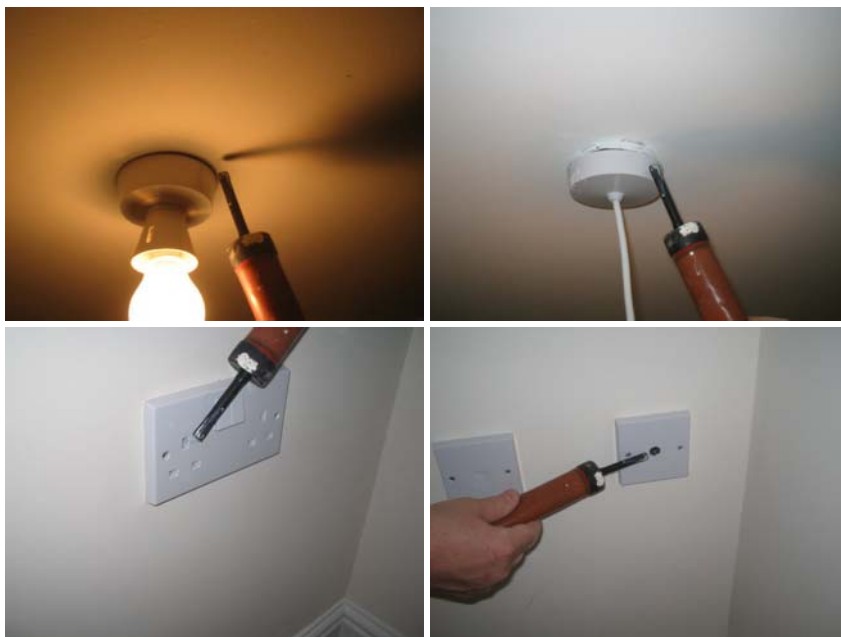
Figure 10.12 Air leakage into the intermediate floor void around central light fittings in the bathroom and a bedroom, and through wall penetrations in a bedroom and the lounge.
