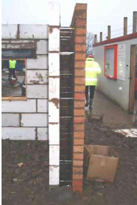
Figure 4: Test wall showing 142mm cavity and plastic ties.
