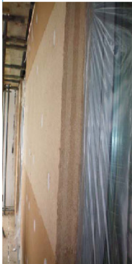
Figures: Fixing the wood-fibre board and the thermally broken fasteners
