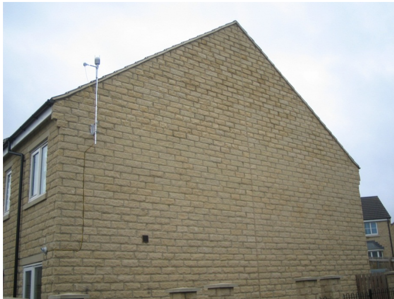
Figure 9 Coheating test weather station installed on a gable wall.
