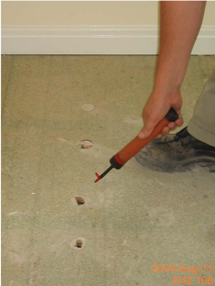
Figure 20 Holes in the flooring panels.
