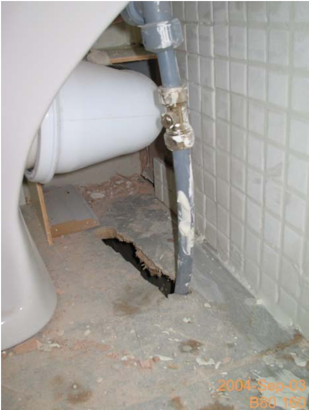
Figure 13 Unsealed service penetrations around WC.
