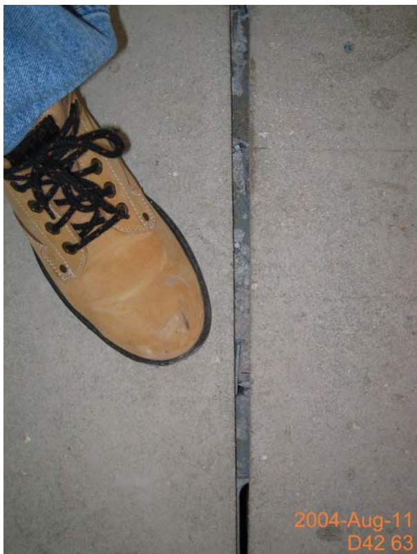
Figure 18 Leaks at the junction between flooring panels.
