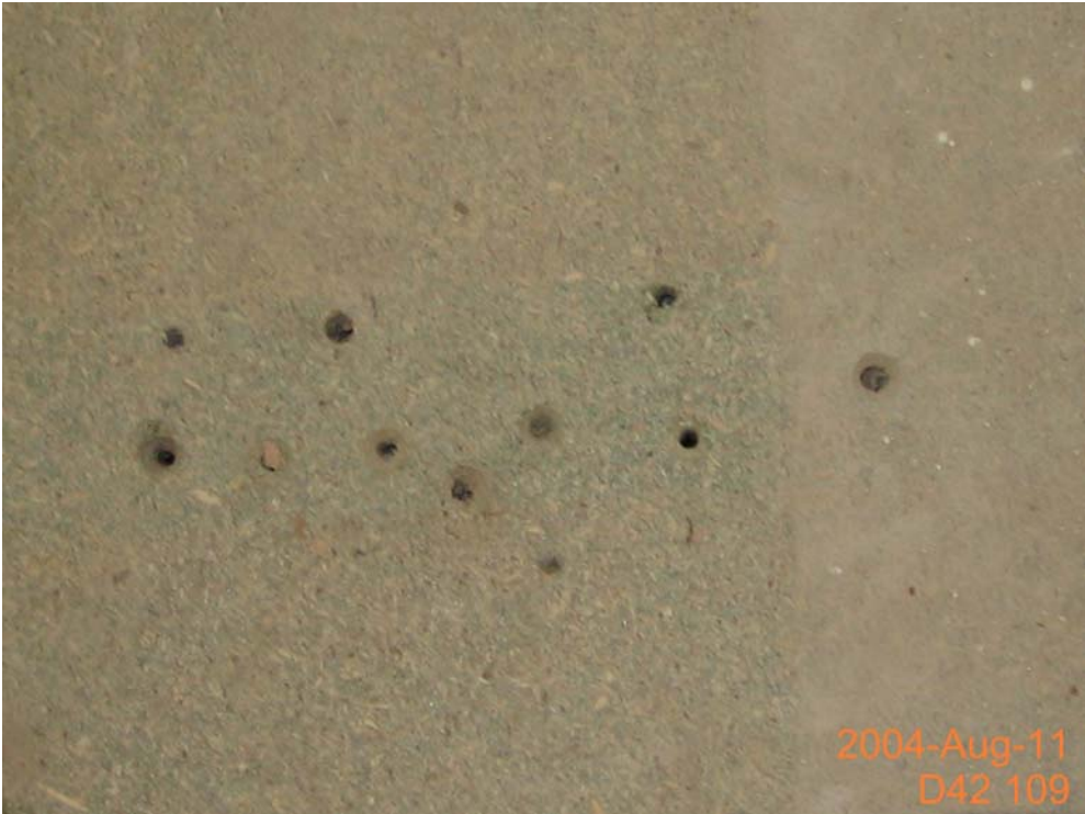
Figure 21 Screw holes in the flooring panels.
