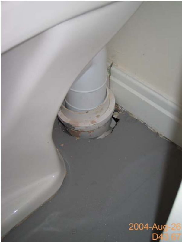
Figure 13 Unsealed service penetrations around WC.
