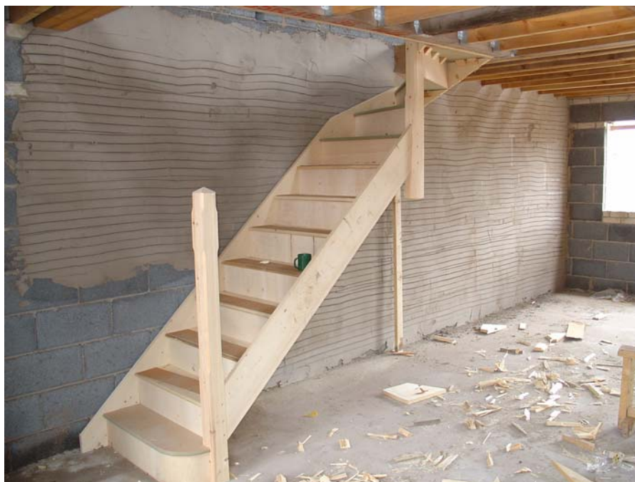
Figure 7 Incomplete scratch coat applied to party walls around stairs.
