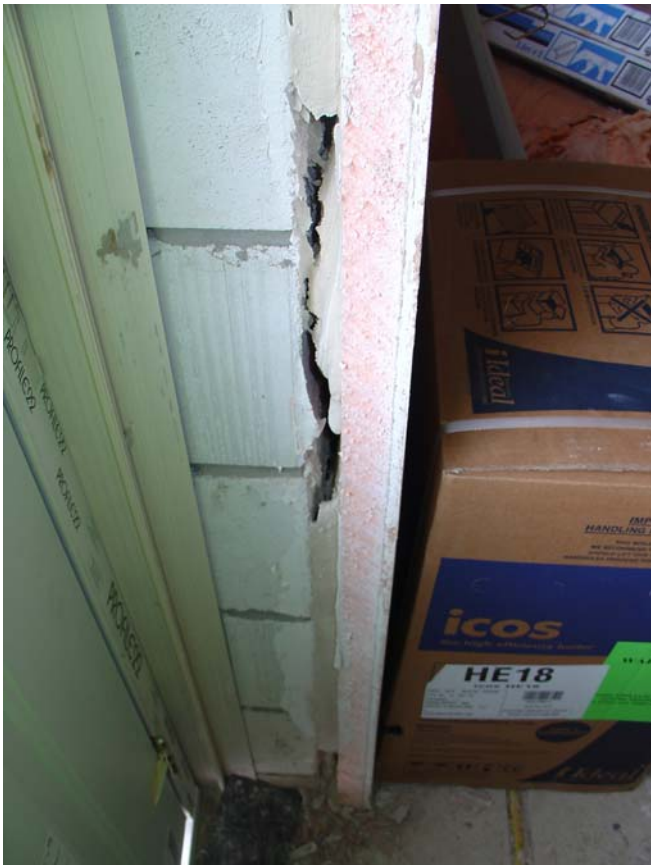
Figure 11 Discontinuous ribbons of adhesive around door opening.
