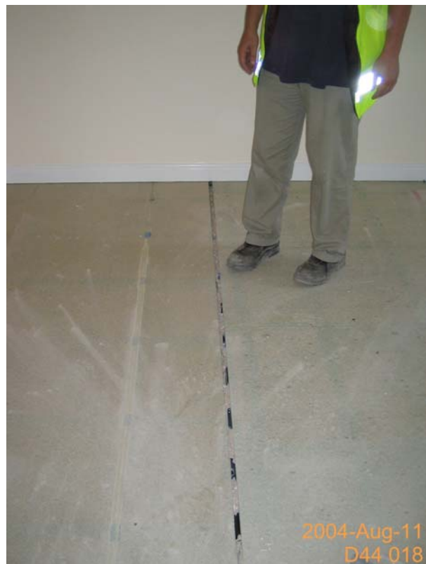
Figure 18 Leaks at the junction between flooring panels.
