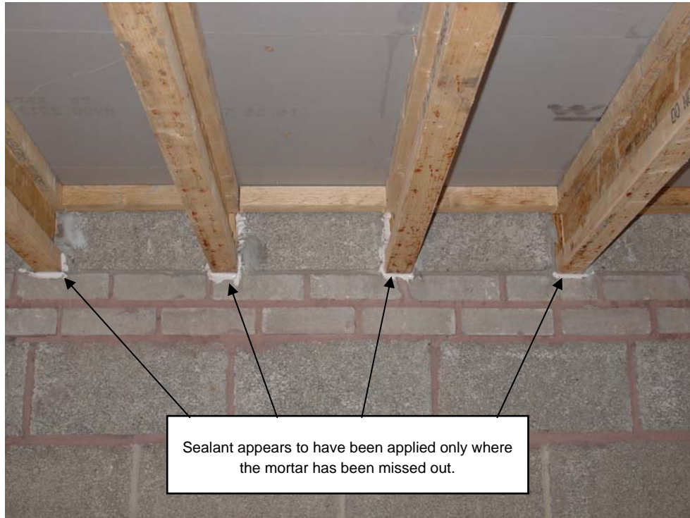
Figure 2 Partial application of mastic sealant (developer B).
