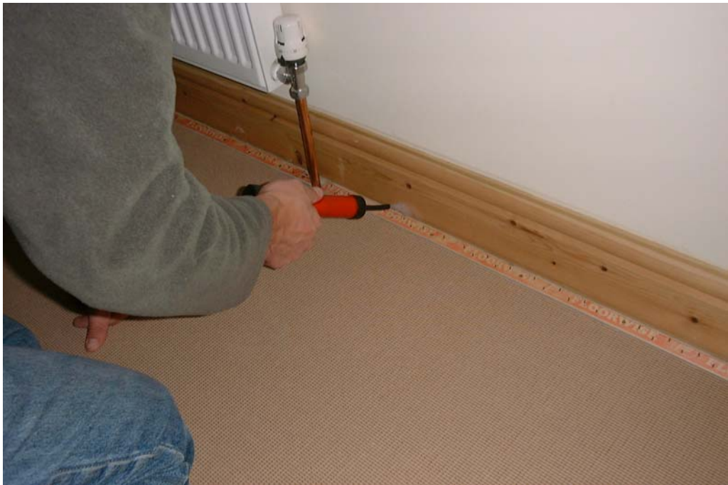
Figure B5 Leakage at the external wall/upper floor junction.
